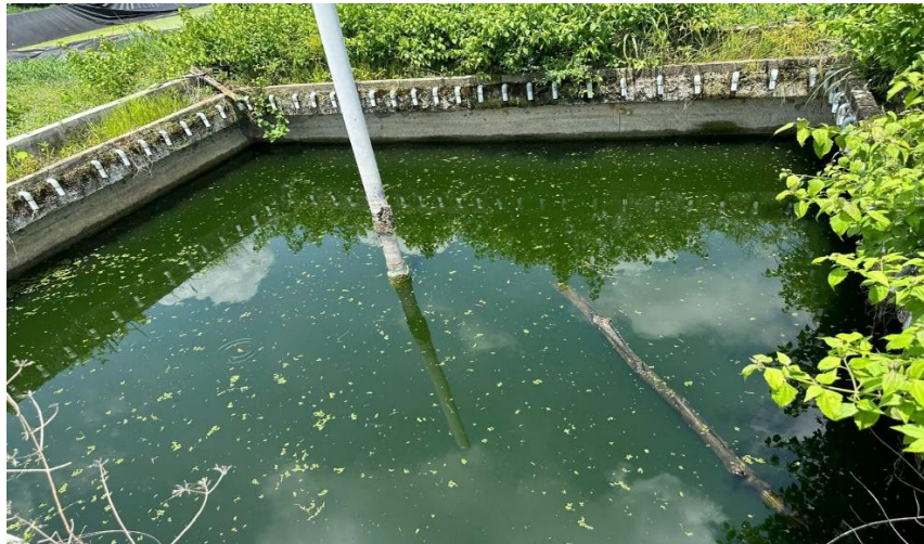
BỂ TRUNG GIAN
